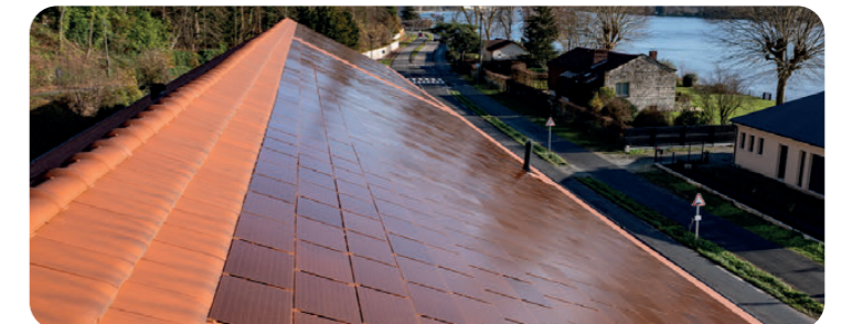
> Roof slope facing due south
