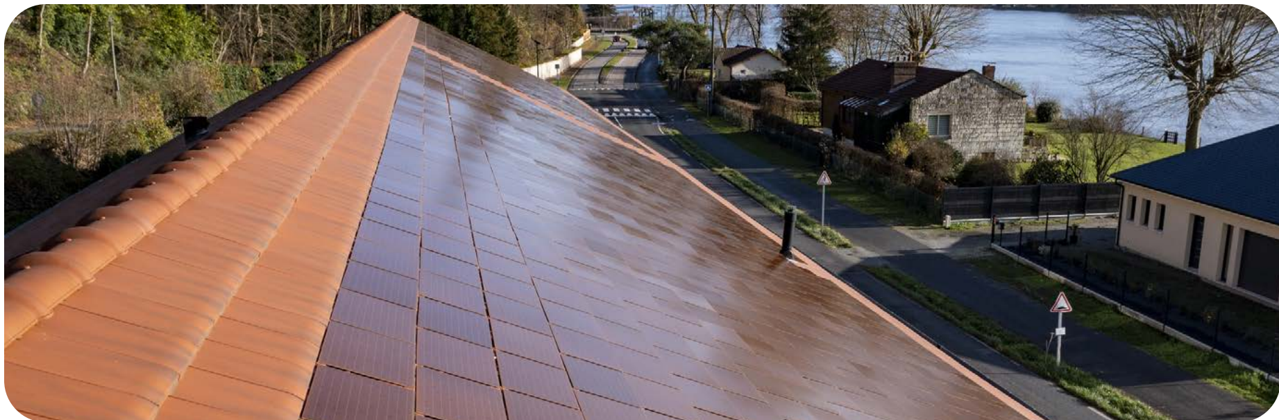
> Roof slope facing due south
